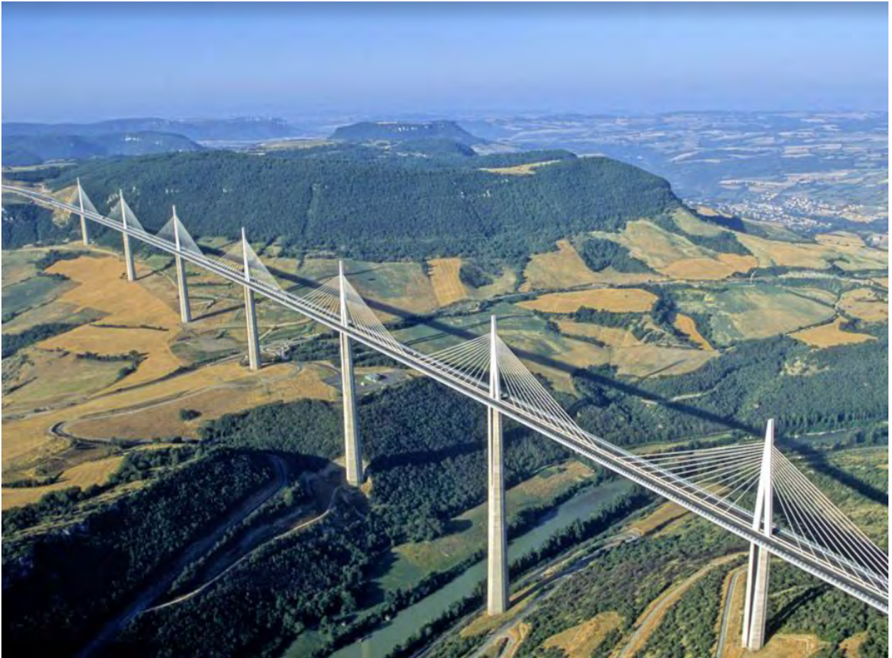
FIGURE 3.1 – Perspective view of the Millau Viaduct
