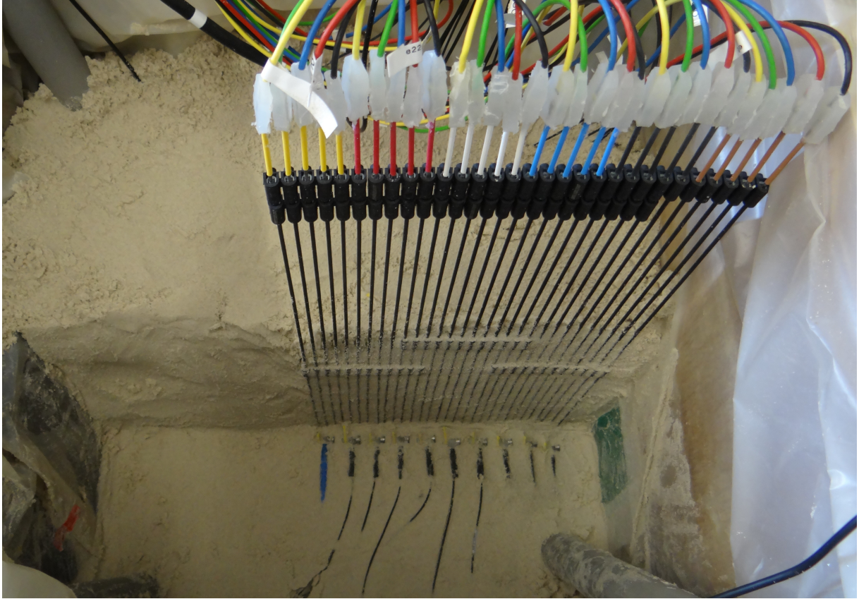
Figure 3.4: Partial emptying of the sandbox after measuring campaign: half of the measuring plane is visible while the other half is covered by a 25 cm thick sand-layer. Rigidifying blocks are placed well off the measuring plane.
