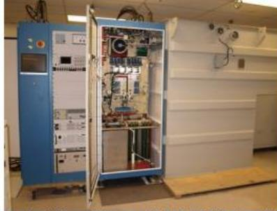
Figure 1. DTI's prototype solid-state ESS-class klystron modulator, developed under a DOE SBIR grant. This design is optimized for long pulse operation with highest possible reliability and availability required for particle accelerator user facilities and test stands.
