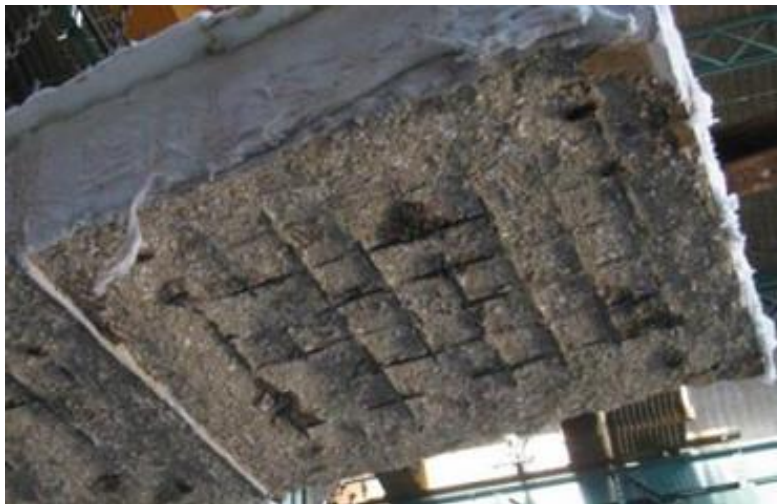
Figure 2.4: The exposed face of the slab after 2 hours of heating.
