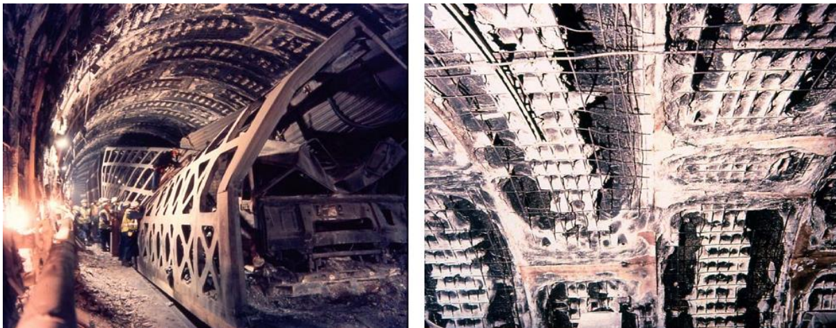
Figure 1.1: Damage in the lining of the Channel Tunnel between France and England after the fire accident on November, 18 th 1996.
