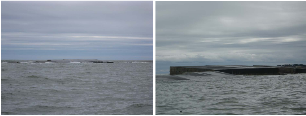
Figure 1.7: Caisson displaced in the offshore breakwater of the Port of Soma (from Tsimopoulou (2011) ).
