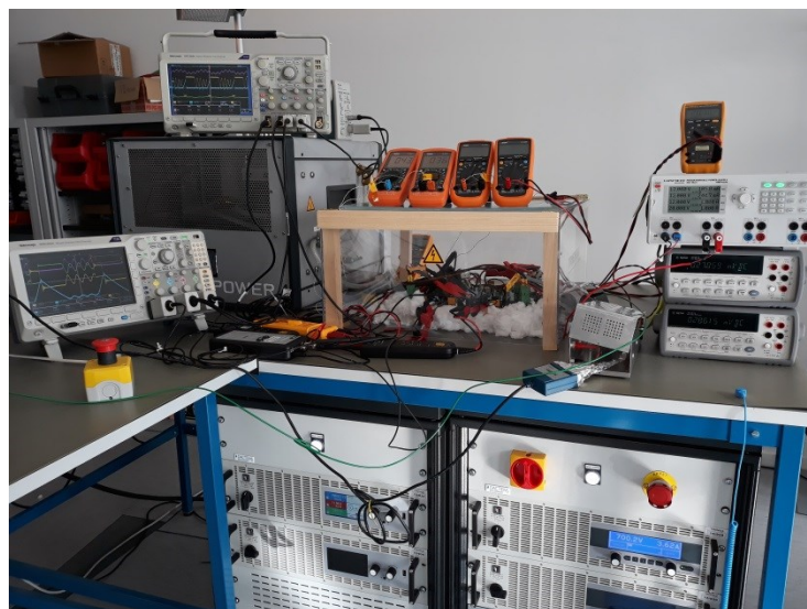
Figure 5: Electrical power test bench: (a) schematic, (b) picture
