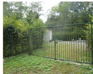
Cesson (77) - Station d'épuration
