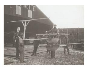
Figure 1.4 - One of the first flight simulators in the world - 1910 - France
