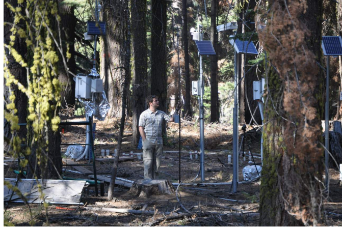
Figure 4.12: A cluster of 5 sensor stations in the the Southern Sierra CZO deployment. Other similar cluster make up this approximately 2 km long deployment.
