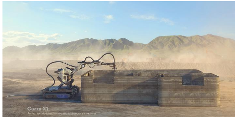
Figure 2.20 – Cazza 3D Robot-based Construction Printer
