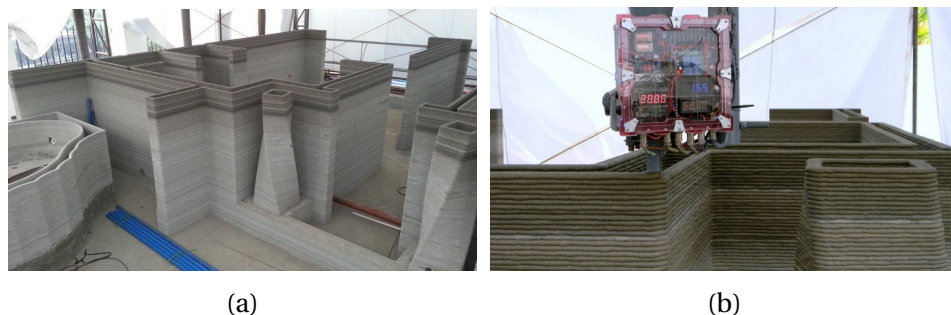
Figure 2.13 – Lewis Grand Hotel extension
