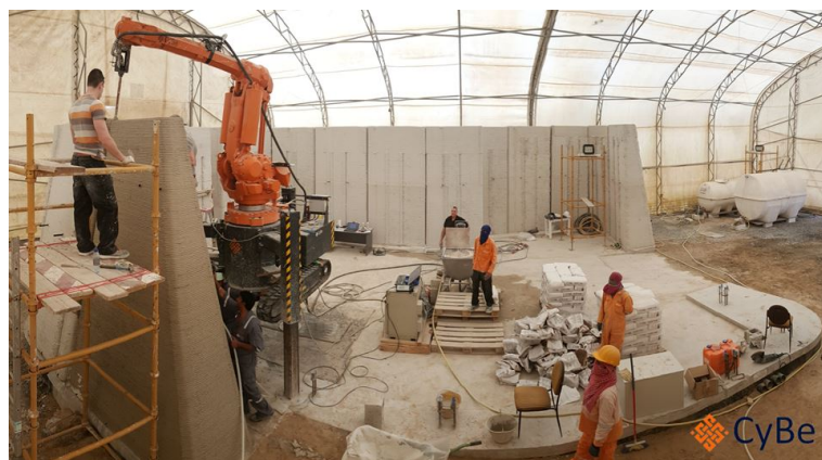
Figure 2.17 – CyBe RC 3Dp mobile 3D printing robot
