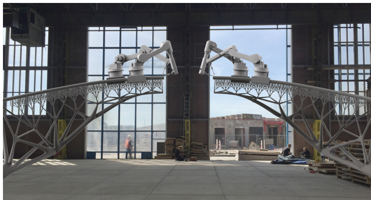
Figure 2.15 – Project of a steel bridge printed in 3D
