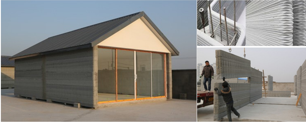
Figure 2.4 – Housing Construction with prefabricated elements using additive manufacturing
