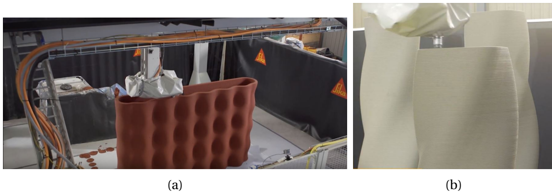
Figure 2.14 – Concrete printing Sika 3D
