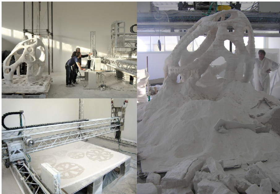
Figure 2.2 – D-Shape : Solidification from sand
