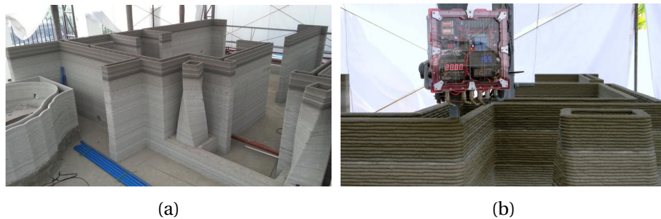
Figure 2.13 – Lewis Grand Hotel extension
