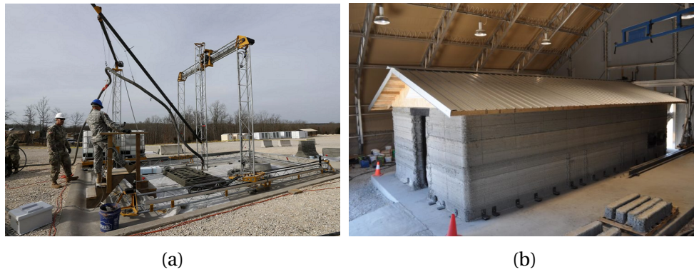
Figure 2.11 – Barracks building printed from local concrete by the US Army
