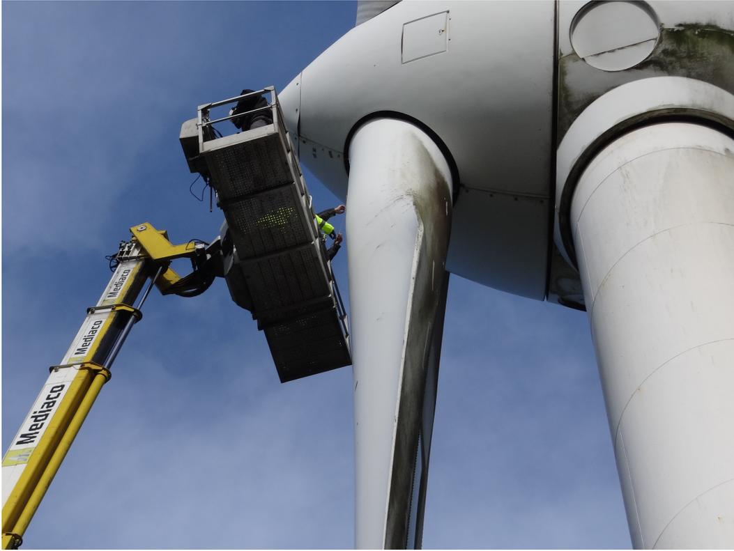
**Figure 4.10:** Aerial work platform positioning
