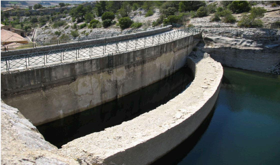
Figure 8. 3 View of the two dams.
