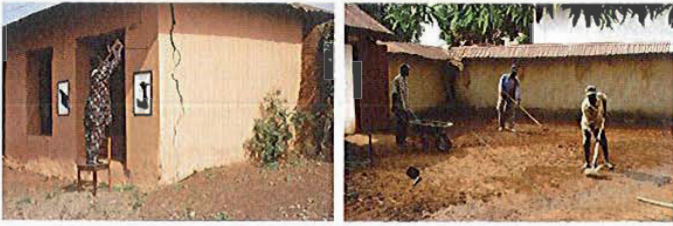
Fig.1 and fig.2 Preventive measures at the Royal Palaces of Abomey, 1996, Prema Project, ICCROM, CRAterre, DPC Benin (credits: Thierry Joffroy, 1996)
