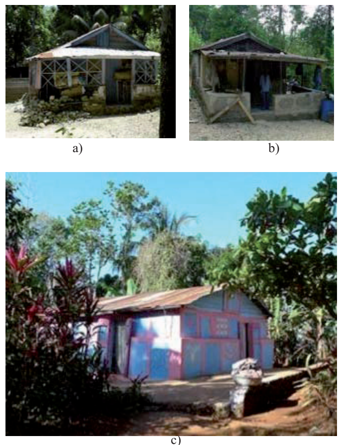
Figure 2. Grande Rivière: (a) disconnection of the gallery structure, (b) bracing of the gallery and decorative frieze (c) Cap Rouge: reduced height and plant barrier to protect against strong winds (credits: Annalisa Caimi).
