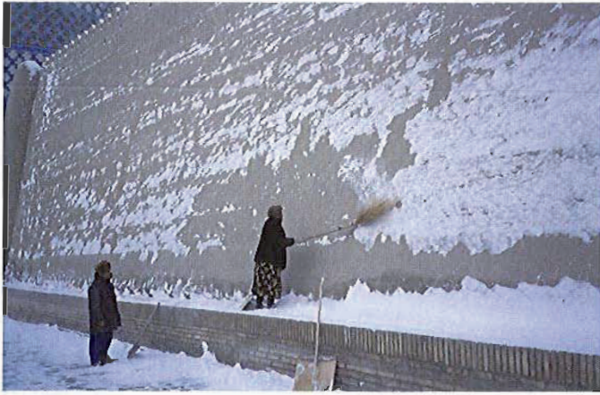
Fig.4 Traditional preventive measure of snow removal from a wall and wall base in Khiva, Uzbekistan (credits: Thierry Joffroy, 2003)
