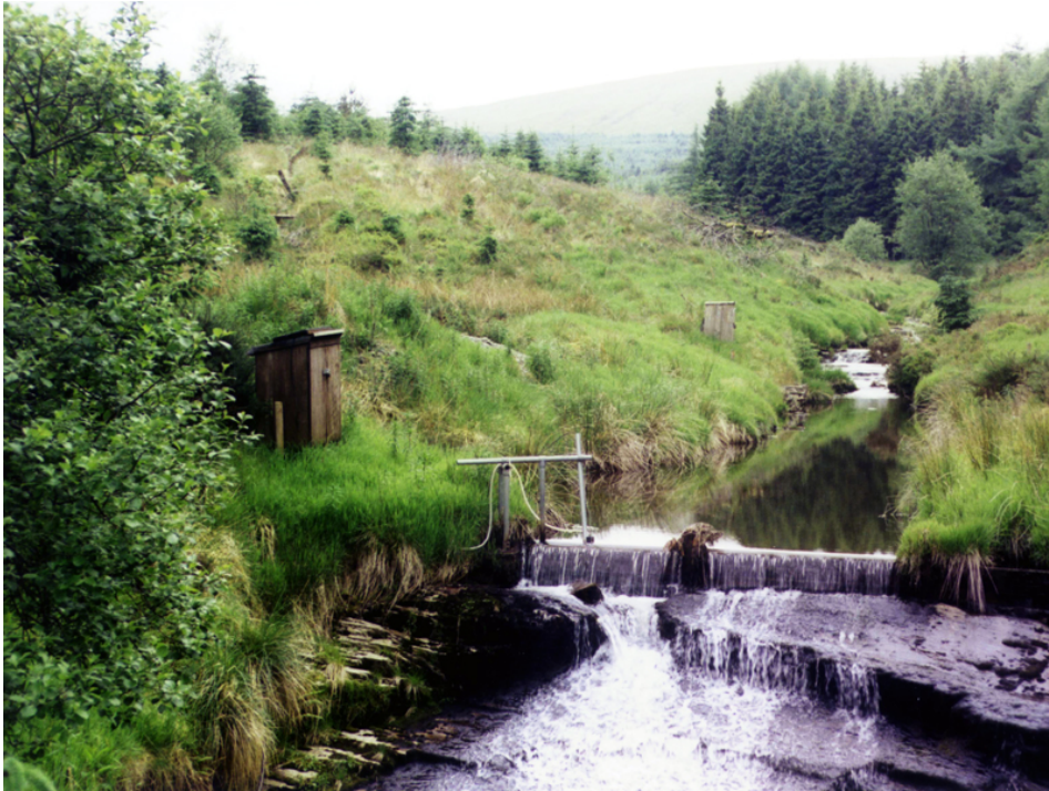
Figure 7.1: A gauging station of the Severn river, Wales ( picture : J. Kirchner, from http://www.ethlife.ethz.ch/archive_articles/130812_Wasserqualitaet_aj/index_EN ).
