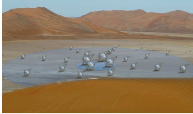
Figure 2.9: Artist's view of a possible layout for the CTA observatory: three classes of telescopes (large, medium and small) will allow to cover a wide energy range from 10 GeV to 200 TeV.
