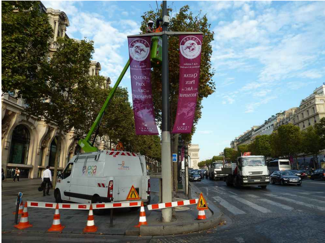
Figure 4.11 – Cradle and workmen installing beacon B_2 on a streetlight pole on the Champs Élysées.
