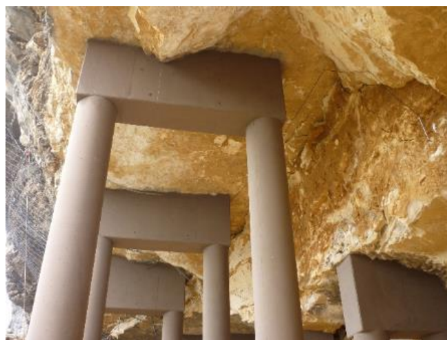
Figure 2-12 Supporting structures inside the cavern
