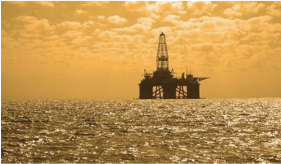
FIGURE 2.1 – Forage pétrolier en mer
