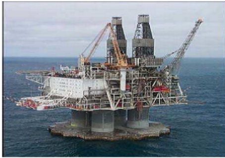
Installation marine (offshore)
