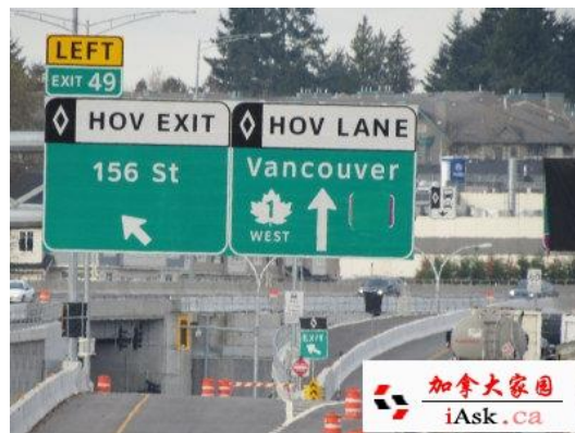
Fig. 2.3 Example of HOV lane in a city
