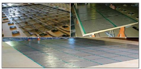
Figure 2.17 – The Sub-floor steel framework (top left), the surface floor wooden framework (top right), the complete view of AME Floor-III after assembly (bottom).
