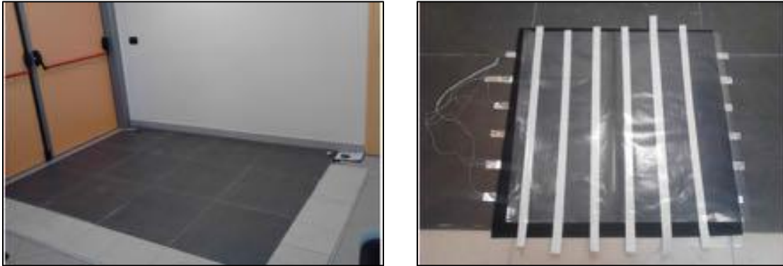
(a) The installed floor prototype
