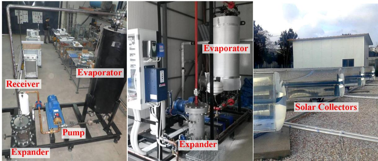
Figure III-3: CPV-Rankine installation pictures
