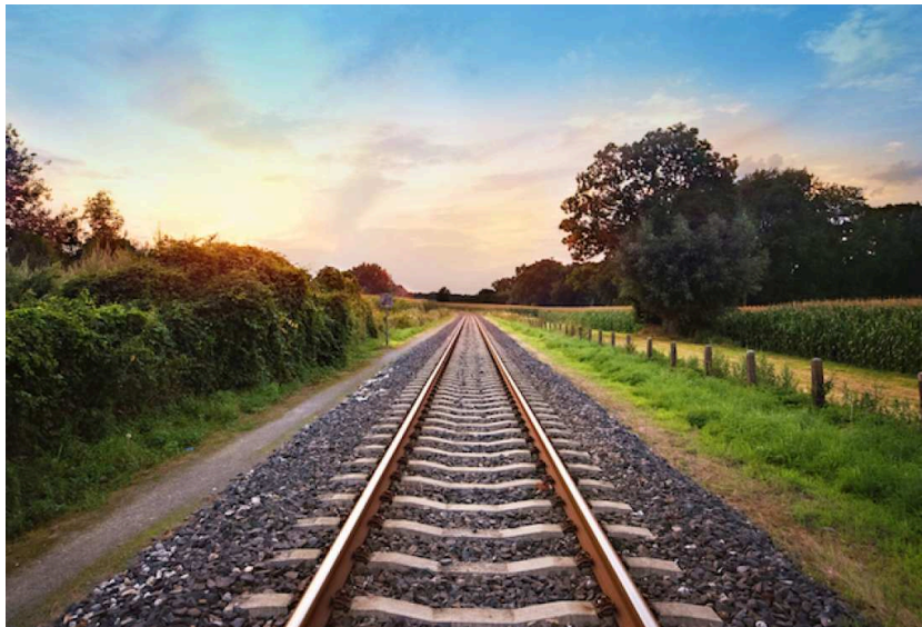
Figure 2.2 Track composed of rails, ties and ballast.
