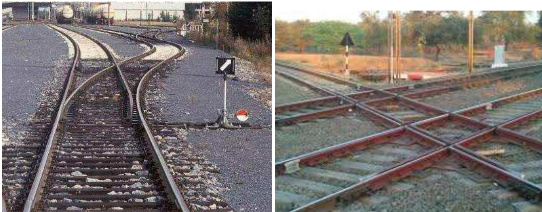
Figure 2.3 A switch on the left, a crossing on the right.
