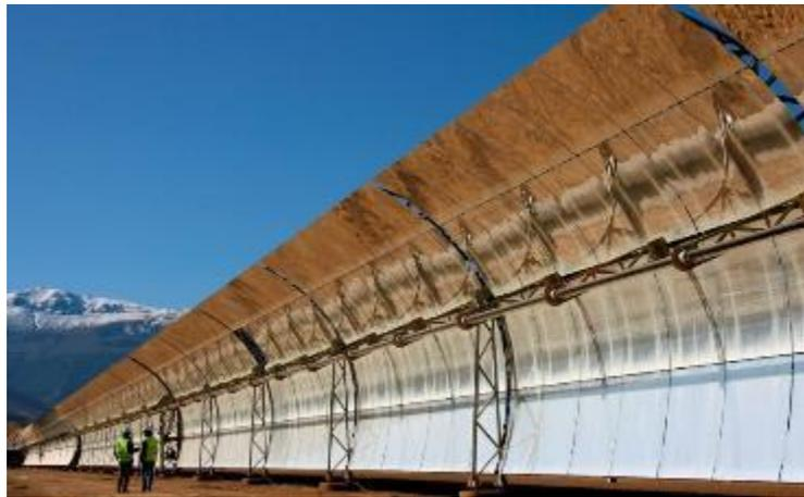
*Figure 1: Centrale CSP cylindro-parabolique Andasol, Espagne (150MWe)*
