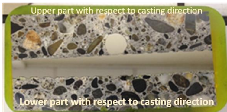
Figure 2-52: sample obtained from a concrete slab
