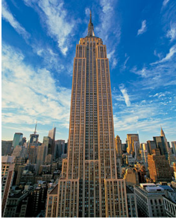
Figure 3.2: The large scales of the Empire State Building.
