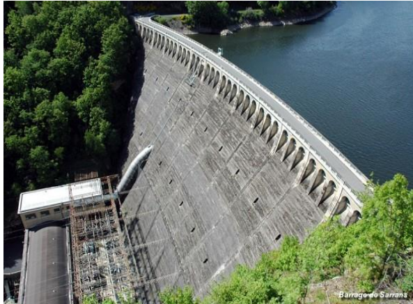
Figure I- 1 Barrage-poids de Sarrans-France ( http://structurae.info/ )
