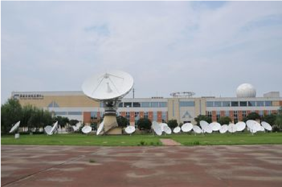
Fig. 1-1 Wireless signal monitoring center
