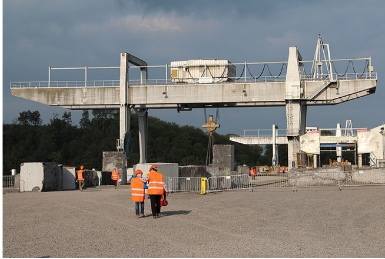
Figure 1.3: Example of an overhead crane in a quarry in Belgium. – Credits: Jean-Pol GRANDMONT (CC-BY 3.0) 2013.
