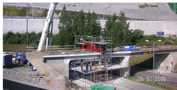
Figure 3.27: Loading setup of the Ornskoldsvik bridge.
