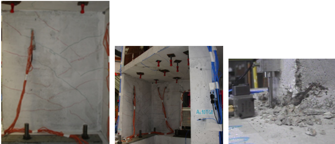
(a) Cracking in shear wall #4 after run #17. (b) Cracking at the 1 st level after run #19. (c) Concrete crushing at the junction between shear wall #4 and the foundation during run #19.
