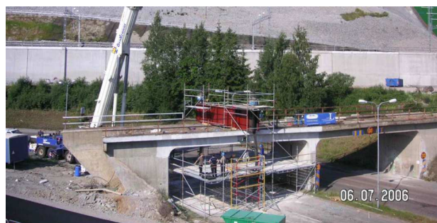
Figure 3.27: Loading setup of the Ornskoldsvik bridge.
