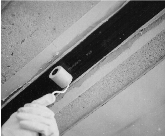
Figure 1.13: FRP strip installation. Reprinted from [4]
