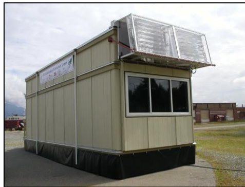
Figure 7 : Solar Canopy Illumination System (Rosemann, Mossman, and Whitehead 2008)
