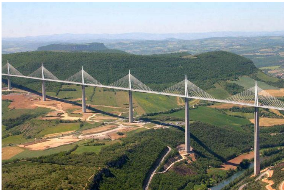
Millau Viaduct: Millau, Midi-Pyrénées, France (HighestBridges.com, 2015)
