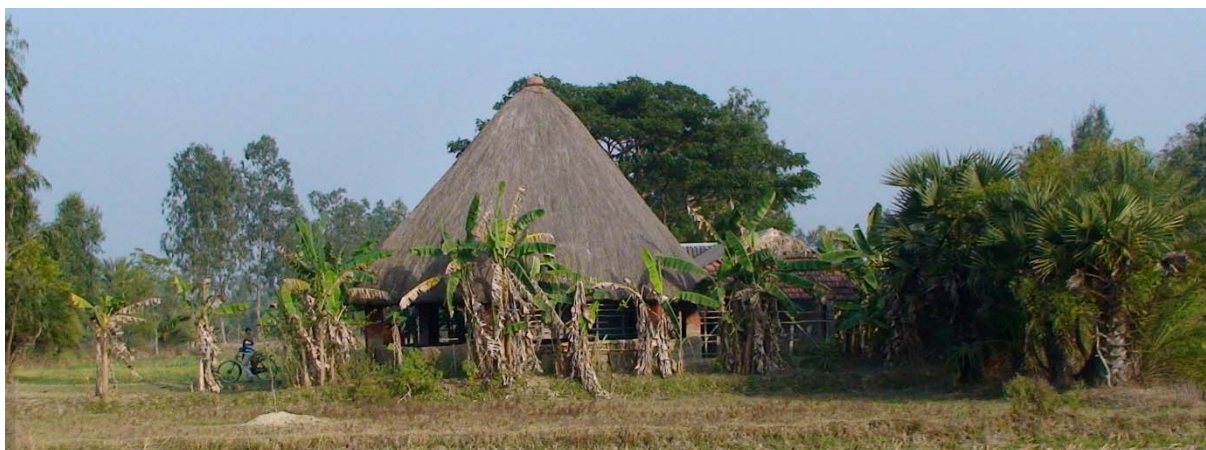
Figure 20 : Mukta Manch de Srinarayanpur
