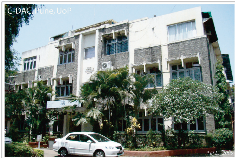
Photo 6.2 – C-DAC Pune, Head Office
