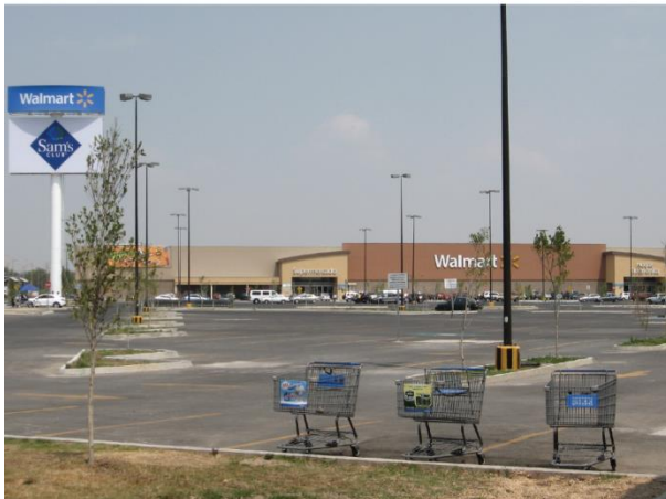
Photo 9.3. Centre commercial, Santa Elena, Cuautitlán, E.de México [2010]
