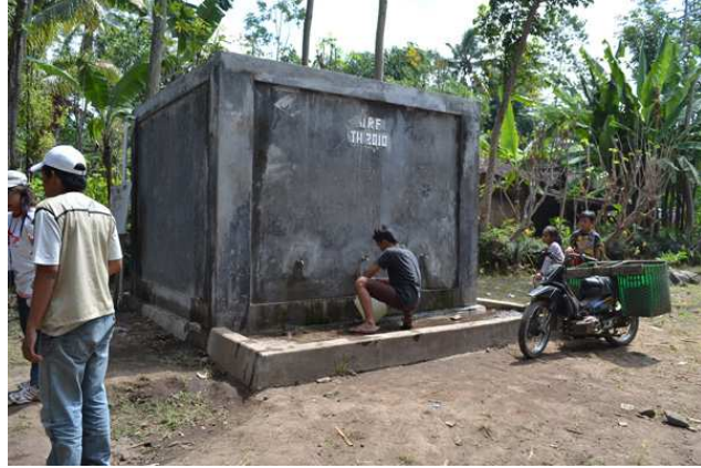
Figure 1.20: Water tank in rural area used for rain water storage during the rainy season and distribution during the dry season.
