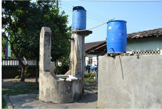
Figure 4.7: Dug well near 450 m elevation (23 m deep).
