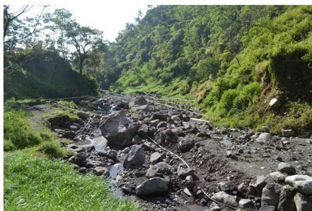
Figure D.4: At Bulu Kidul spring, the famers have installed PVC pipe directly into the river bed to catch the top of the paleo-channel aquifer. The river shows a low surface flow here but 500 m downstream, the river bed is completely under water.
