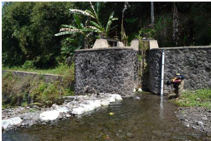
Figure 3.5: Automatic Water level recorder (AWLR) on the Pusur river at Kemiri dam (400 m asl). The floating system is protected from the solid discharge by a PVC tube (in white) and fixed on the dam's wall.
