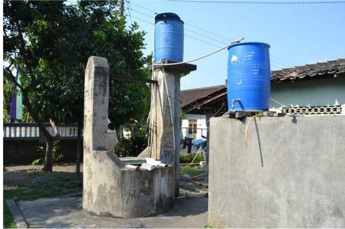
Figure 4.7: Dug well near 450 m elevation (23 m deep).
