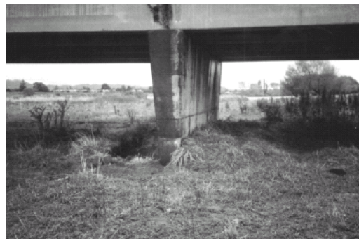
Figure 2.18: Pier C. The mound of the soil on the one side of the pier and the gap on the riverward side (after Berrill et al. [8])
