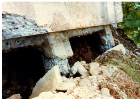
Figure 2.7: Rio Banano Bridge: Front raked piles were more heavily damaged than the rear vertical piles after the 1991 Costa Rica Earthquake (after Priestly et al. [5])
