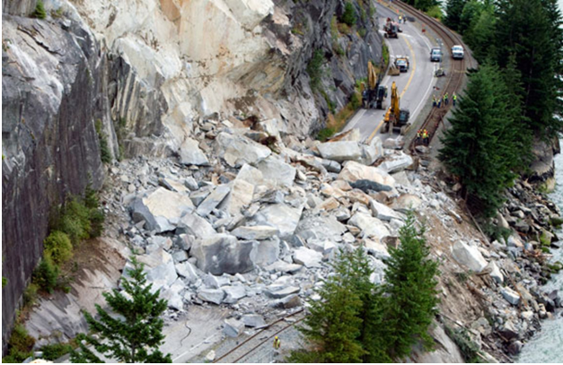
Fig. 1. Rockfall on Sea to Sky highway (B.C.). Note the jointed structure of the source area (Canadian Press photos).
