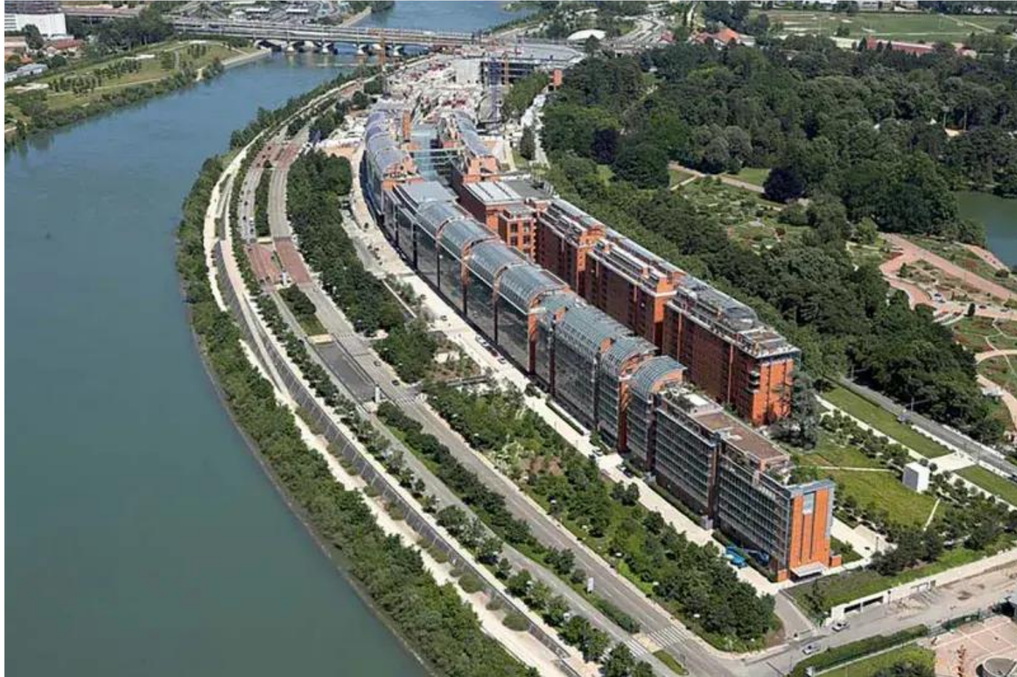
Cité Internationale Renzo Piano Building Workshop (2006) Lyon
