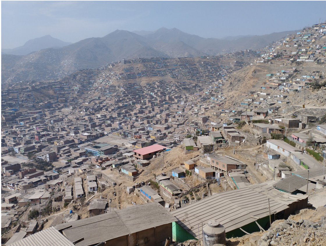
Figure 2. Informal urbanisation on the outlying heights of Lima, in Villa Maria el Triunfo
