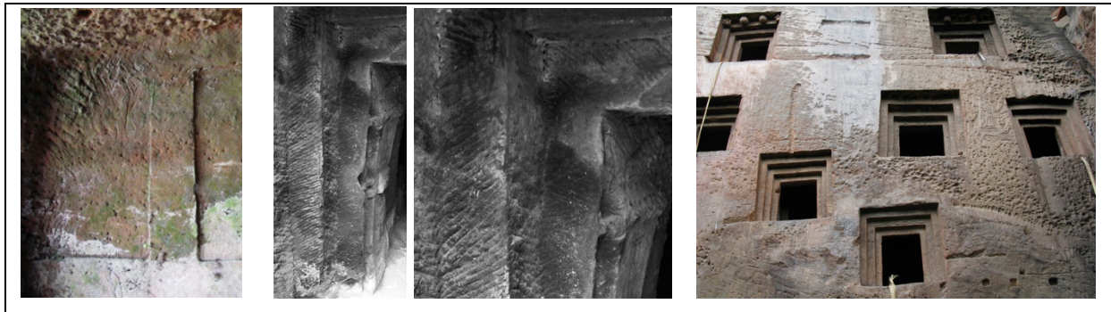
Fig.16.(A).Transition zone between dressing stages. Xiaobao, Chezi district, Leshan city.– (B).Alterned quarried and dressed surfaces. Citangpo M9 stepped door. – (C).Stepped doors. Qigedong, Changning County.
