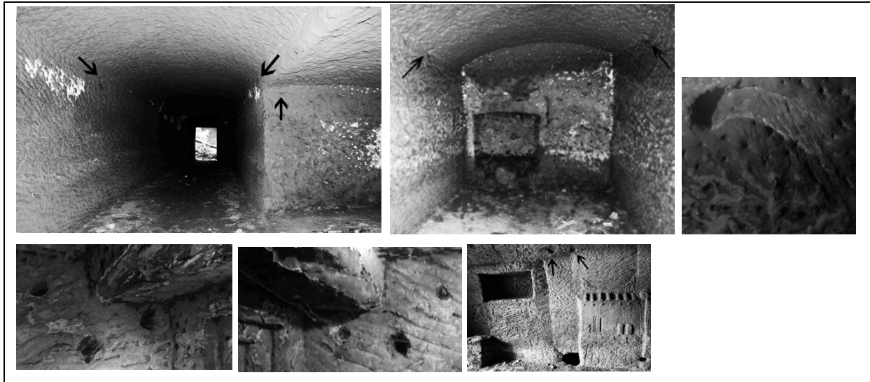
Fig.8.(A-B).Symmetric pair of holes. Xiaoba, Chezi district, Leshan city.(车子镇肖坝). -- (C).Grooved hole. Xiaoba, Chezi district, Leshan city. -- (D-E).Paired series of three holes by a stepped door. Xiaoba, Chezi district, Leshan city.-- (F).Two round holes.Citangpo M9 Left wall.
