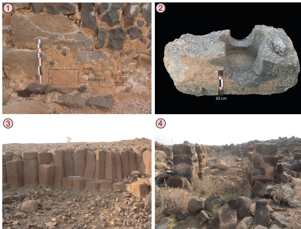
FIGURE 8 | Photographs of the main archaeological features (mapped on Figure 5) discovered during surveys around Sadd al-Bint. (1) Fired bricks found within the mortar of the dam, (2) a stone dam mechanism, (3) possible quarry area along the south bank of the dam and (4) a structure potentially related to the dam.
