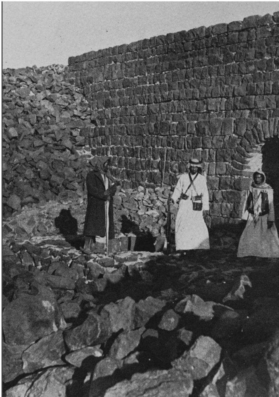
FIGURE 10 | Photograph taken in the 1950s of al-Hasid dam from its downstream side (after Philby 1957). Note the presence of an arched sluice gate at the base of the dam.
