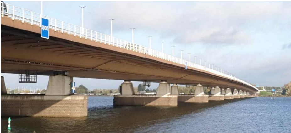
Figure 1. Road bridge structure consisting of ten simply supported steel box girders.
