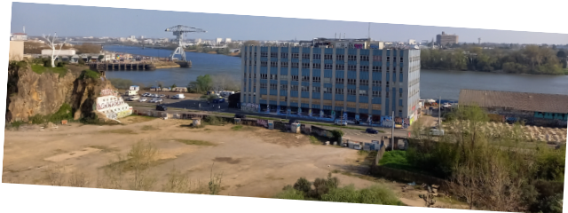
Figure 3: CAP44 before rehabilitation
